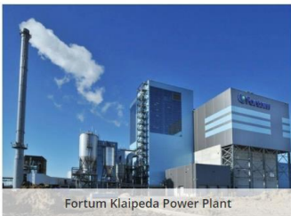
Fortum Klaipeda Power Plant
