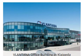
VLANTANA Office Building In Klaipėda
